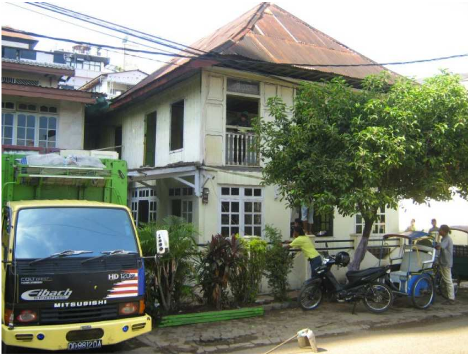
Figure 10.1 Unusu Daeng Remba's house in Jalan Maipa, Makassar, shortly before its demolition on 3 November 2011
